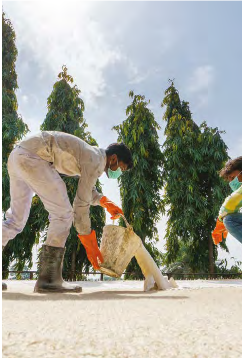
applying the latex
